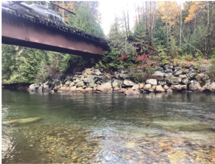
Right Bank Abutment when facing downstream
