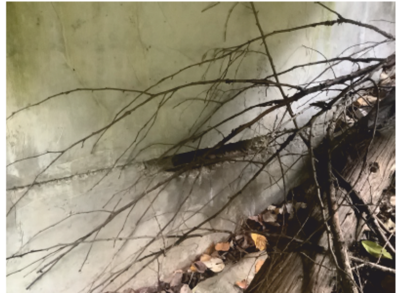
Concrete n right bank abutment
